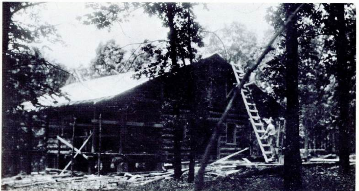
Construction of the first administration lodge was well underway by June 1930. This building today utilized as a Nature Museum in Camp Wigwam of the H. Roe Bartle Scout Reservation.
