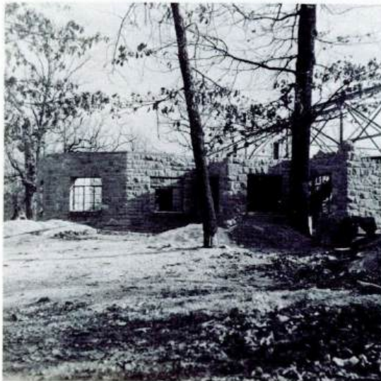
By mid-1950 the distinctive sandstone structure of the Memorial Lodge was halfway completed.
