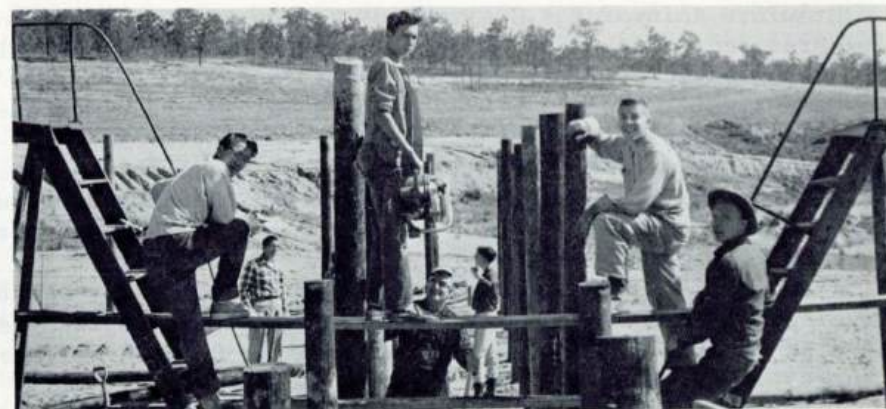
Some early construction at Spanish Trail Scout Reservation.
