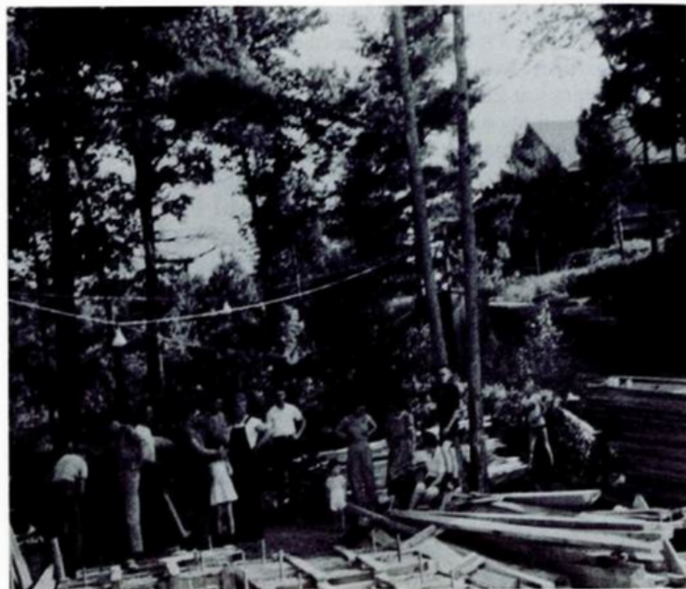
Construction of the first swimming pier at the Camp Carpenter waterfront. The existence of the superior camping facilities in the Daniel Webster Council has always depended on the enthusiastic support of volunteers. Willing Scouters and their friends, under the supervision of professionals and volunteer "experts" have achieved miracles in camp construction projects.
