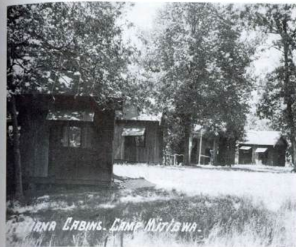
Ojetirna Cabins at Camp Mitigwa.
