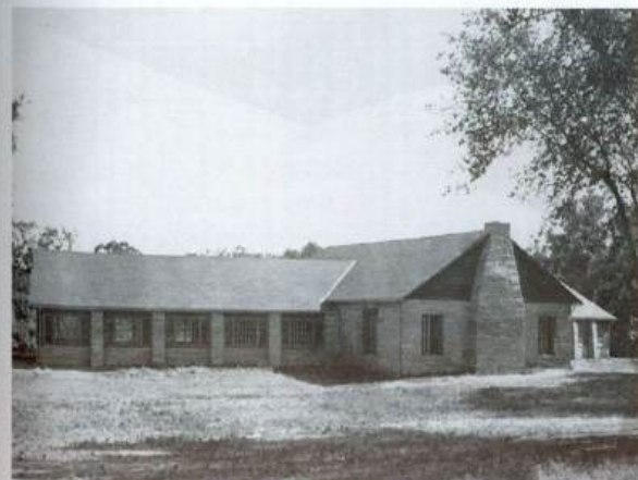
Blank dining hall after reconstruction.
