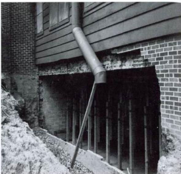
A rear-view of foundation work done on Blank Dining Hall.
