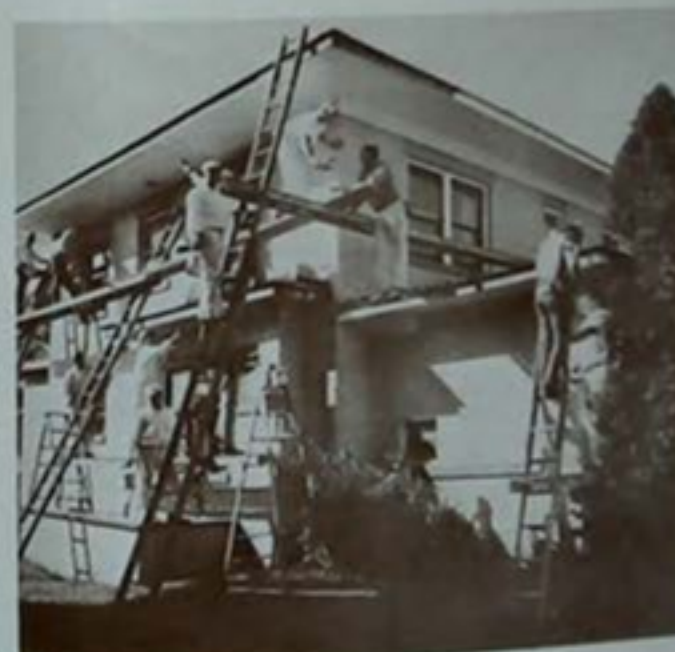
Scout Office remodeling
