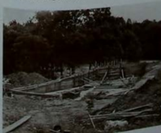
Camp Buckeye pool construction
