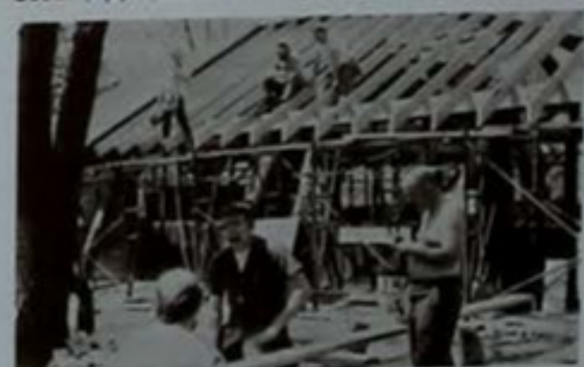
Replacing the dining hall roof
