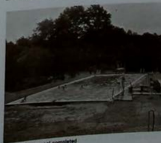
Camp Buckeye pool completed
