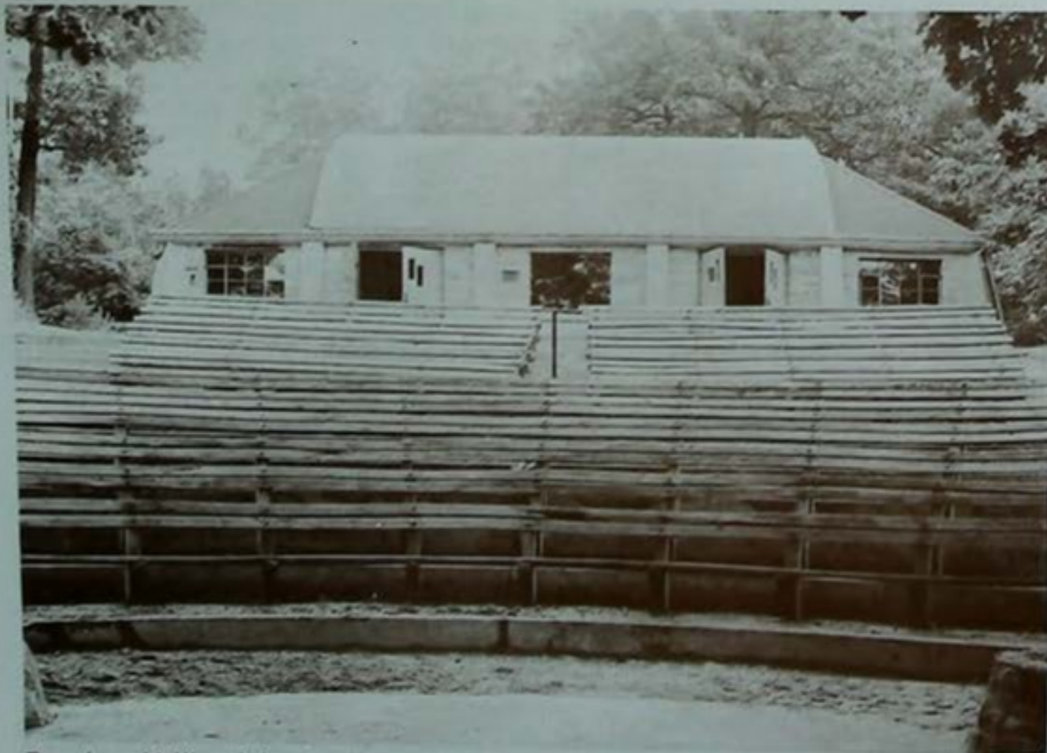
The newly completed Hoover Lodge and amphitheater at Camp Tuscazoar
