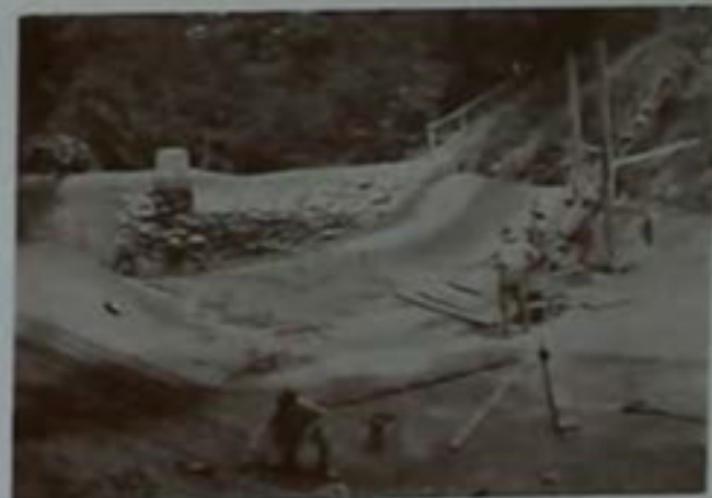
Constructing the first swimming pool
