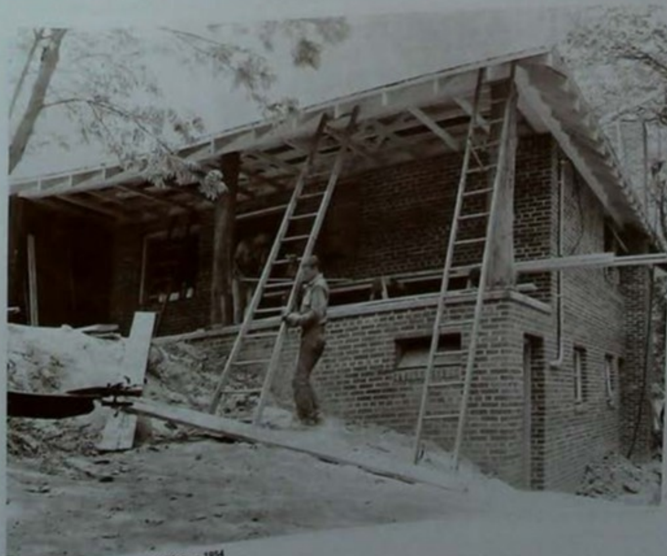
Tuscazoar dining hall kitchen addition — 1954
