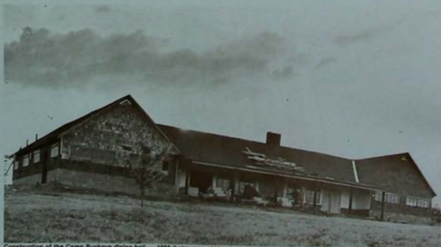
Construction of the Camp Buckeye dining hall — 1955 (Later named Hunsinger Lodge)
