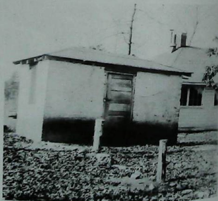
Pump house at Camp Uwharrie located across from the Berlin Lodge.
