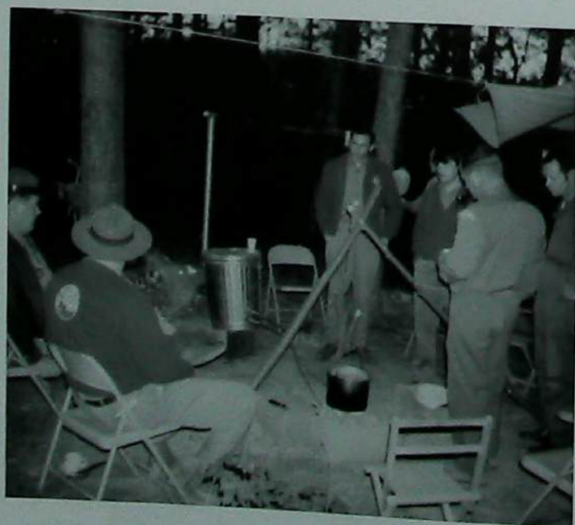
This campsite water heater was a trademark of Bob Bruton, Scoutmaster from Lexington during camping trips and council events in the 1960s and 1970s. The coils were placed in the fire and water was added to the garbage can to provide a continuous supply of hot water.
