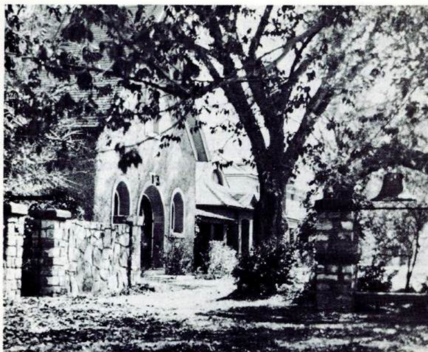
Boy Scout Clubhouse in Roswell. It was used from 1921 through 1925. It was located at 311 N. Pennsylvania.
