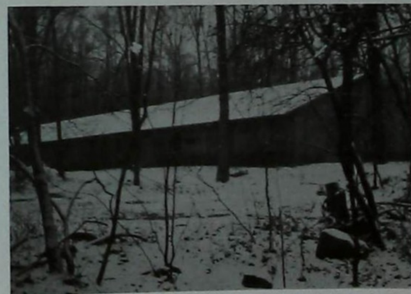
The Gordon D. Bowman Activities Lodge, dedicated in July, 1973. The multipurpose structure measures 40 feet by 144 feet.
