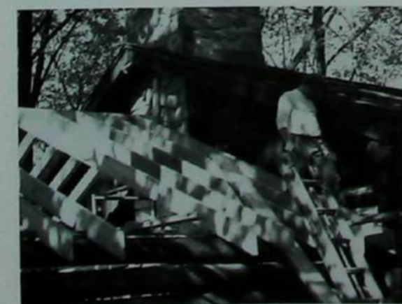
Craig Hadden installing roof rafters
