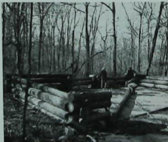
Raising the telephone pole walls, January 1973
