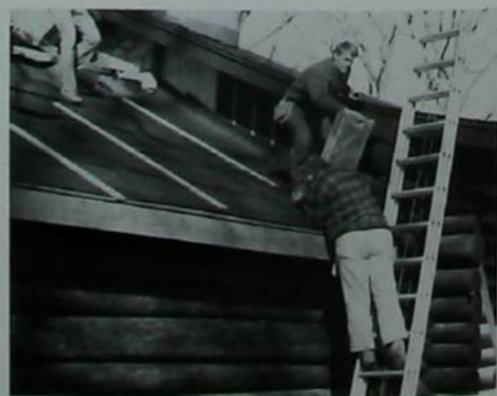
Drew Jordan and Dick Jordan lifting asphalt shingles
