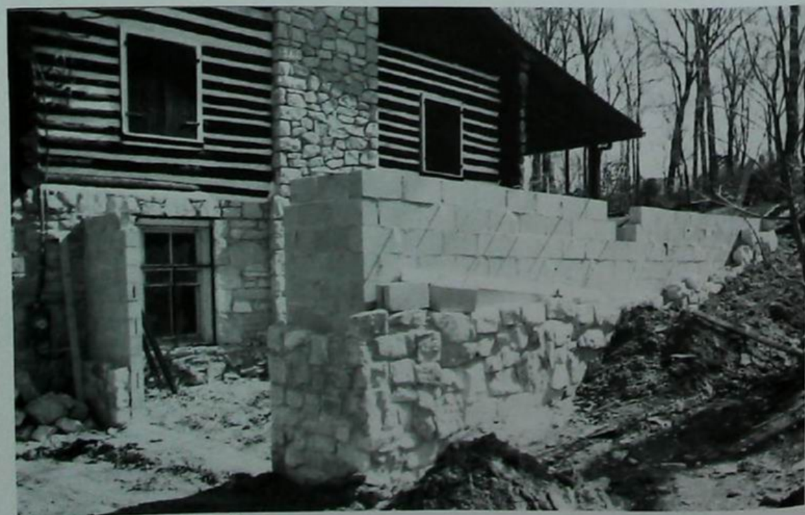
The cinder blocks and stone facing walls
