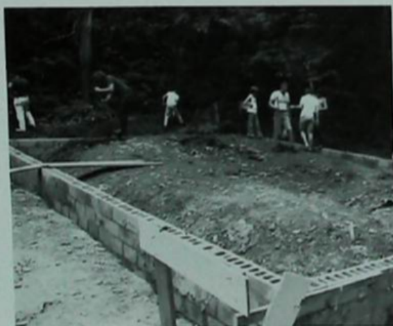
Canoe Barn foundation, June 1972
