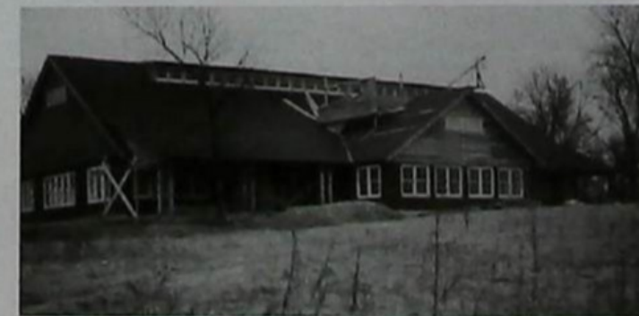
Adding McKinstry Lounge and the porch to the Dining Hall
