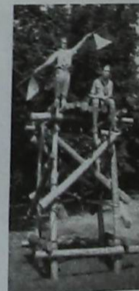
Signal Tower pioneering project at Ingawanis
