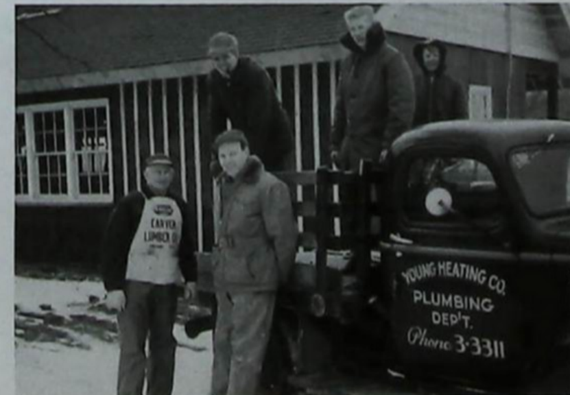
Some of the workers during the construction of the kitchen
