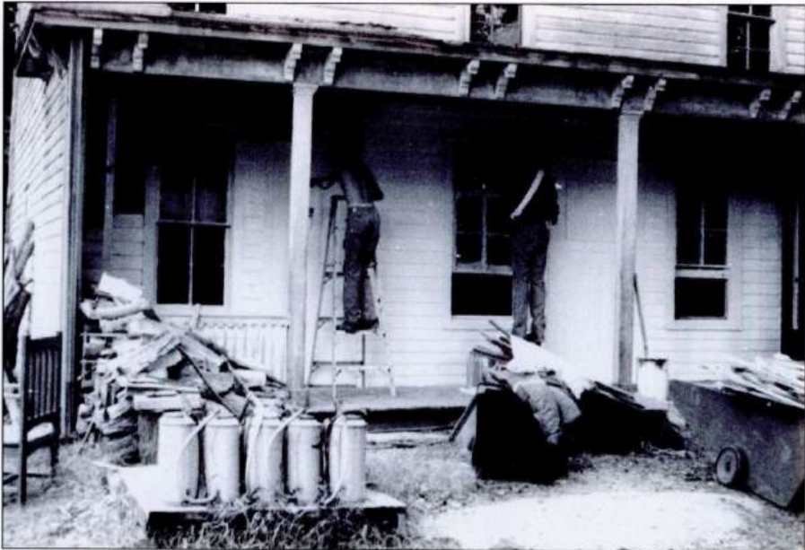
An Order of the Arrow work crew painted the LeValley House during the Order of the Arrow Fall Powwow in 1978. Each year at the powwow, various camp-improvement service projects are accomplished, from cutting brush, painting, and plumbing to maintaining the roads and trails.
