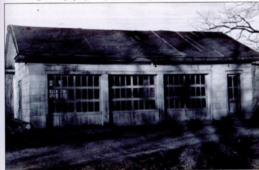
When the LeValley property was converted to be Quail Hill, cots and a wood stove were provided for four-season cabin camping in the garage next to the farmhouse. The author recalls staying in this building in the early 1970s, when it had a very dusty woodchip floor. It was renovated by the Order of the Arrow and named Devlin Lodge in 1978. There is a picture of Thomas Devlin in chapter 8.
