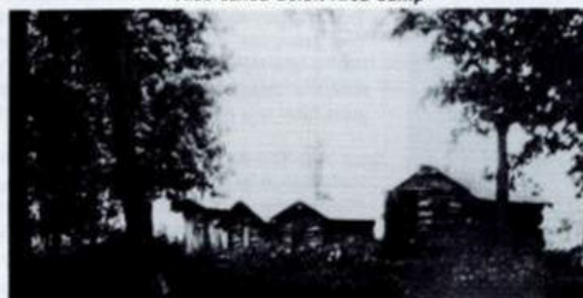
Cabins for camping
