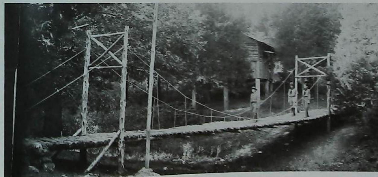
It was safer than it looks. Scouts and staffers built this suspension bridge at Camp Irondale in the early Thirties.
