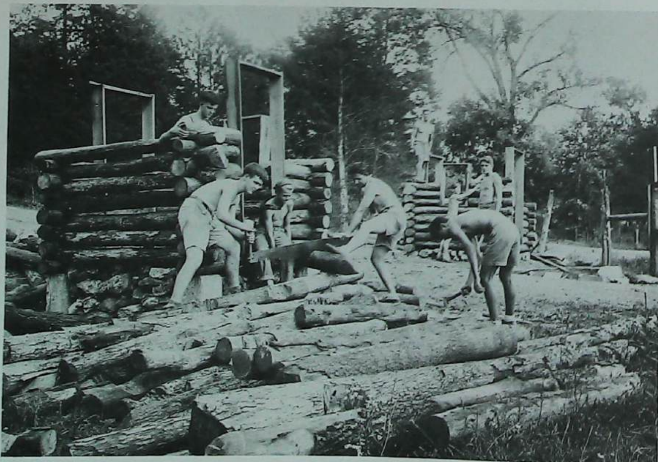
Husky Scouts build the new entrance to Camp Irondale, 1935.
