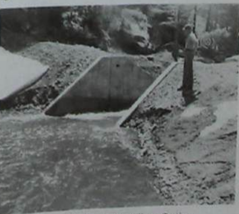
Dam with Removable Spillway Section
