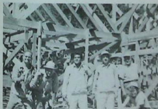
Dining Hall Construction, circa 1950
