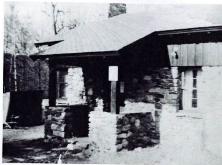
ER Cabin was destroyed by fire. (photo supplied by Harry and Paul Segerstrom)
