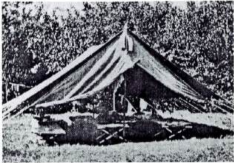
One of the large wall tents at Camp Heinzman
