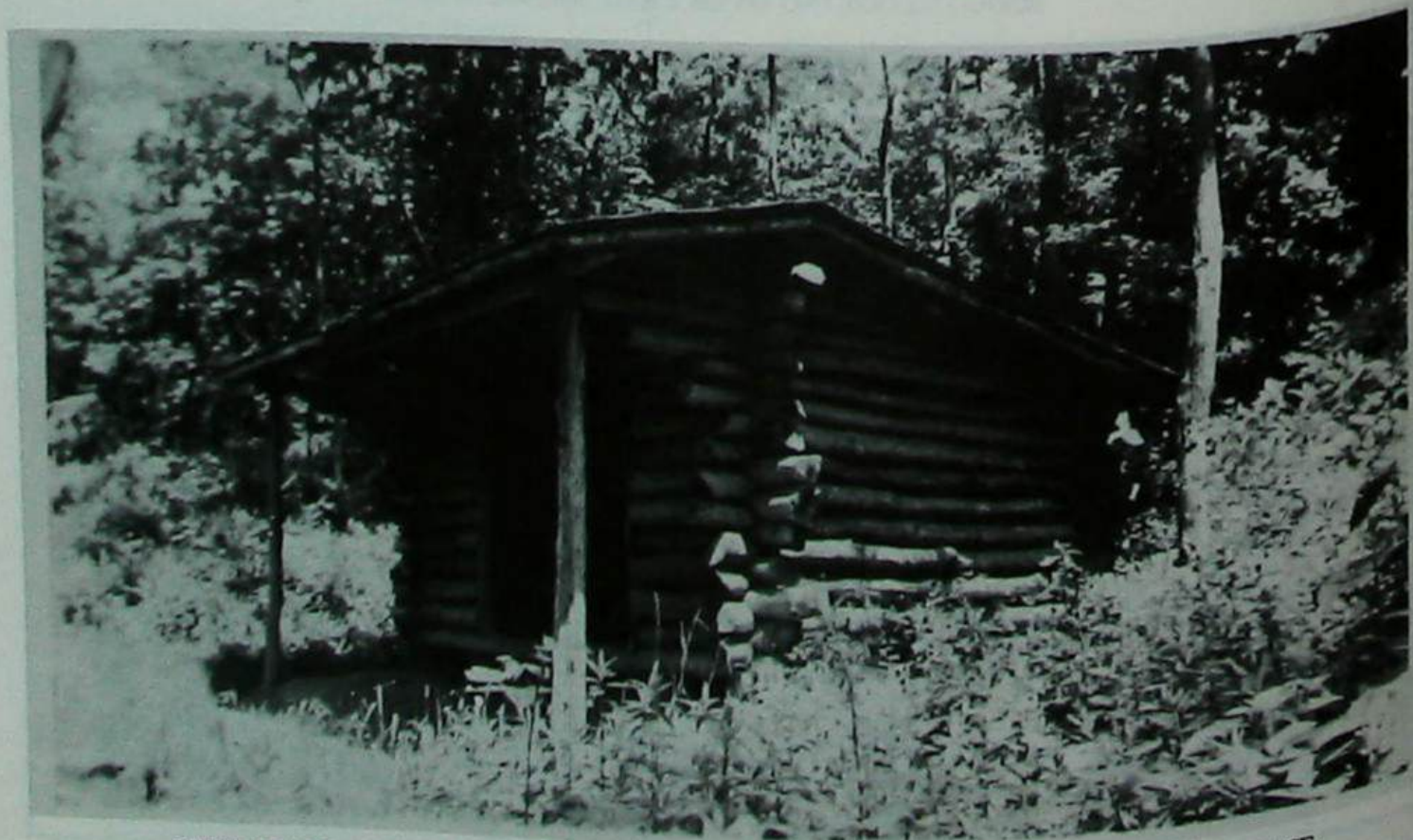
NEW LEAN-TO BUILD ALONG SIDE OF THE LAKE USED BY WATERFRONT STAFF THROUGHOUT THE 1940s
