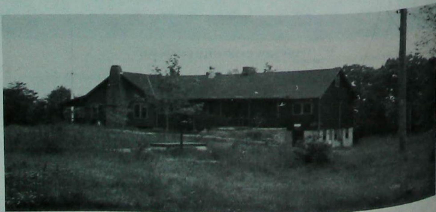
TWO STORY KITCHEN WING ON MESS HALL 1952
