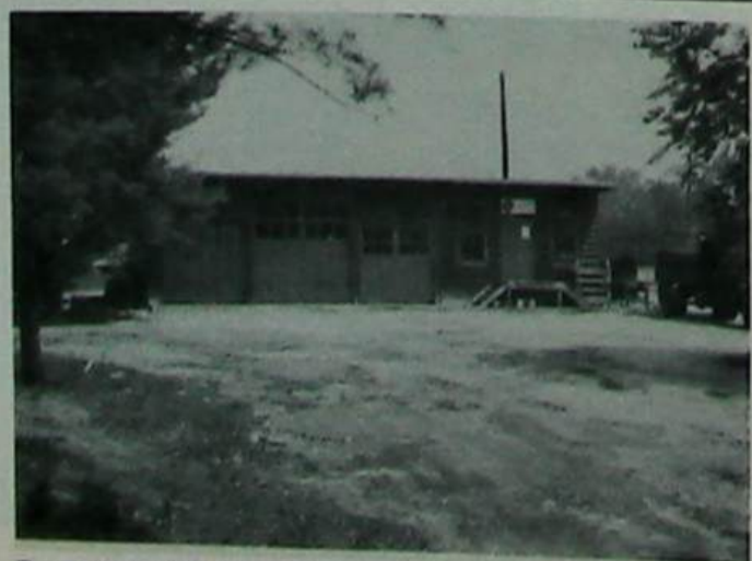
BAITING HOLLOW CAMP GARAGE AND MAINTENANCE SHOP 1949
