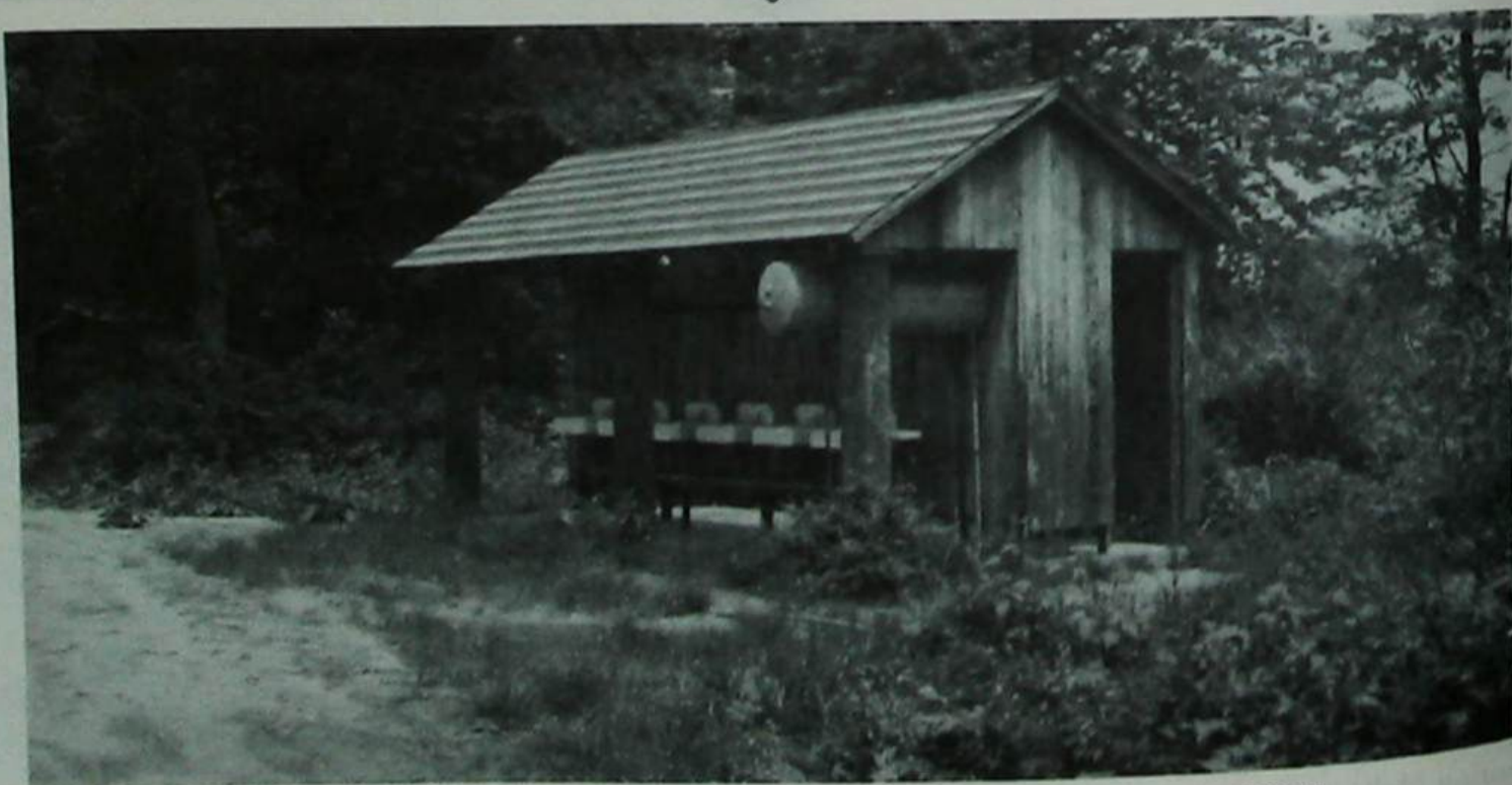
WASH STATION & SHOWER HOUSE AT NATHAN HALE CAMPSITE
