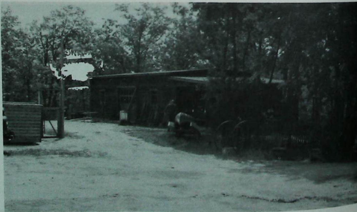
STOREHOUSE AND GARAGE FOR CAMP FIRE TRUCK 1951
