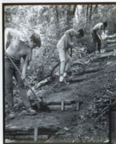
Above - Explorer Post 4 of Camp Hill installs some anti-erosion devices on a trail at Hidden Valley. The work was hard on a hot summer day. Shown are Dave Hull, Paul Howley, and Jim Ruggaber.
