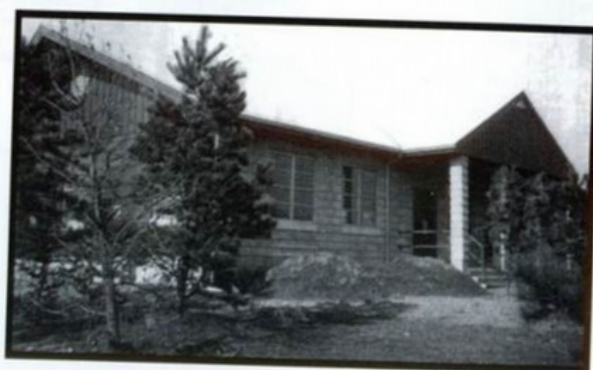
Above - This is Hershey Dining Hall as it looked in 1965. Check out the fresh piles of dirt from new construction.
