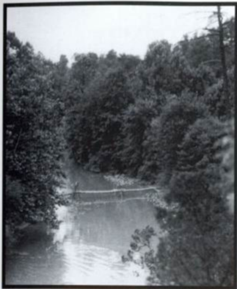
Above - This is a primitive footbridge built over Sherman's Creek. It was used to cross from East to West shore. (O. J. Dickey photo)
