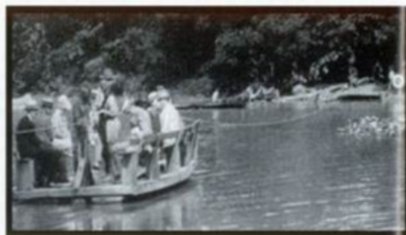
A ferry that crossed Sherman's Creek was the original transportation into Hidden Valley. A stout rope connected both sides of the creek, and the ferry was Scout-powered, pulled by the boys from side to side. The ferry was replaced by a pontoon bridge, and later a wooden-decked steel bridge. Photo by L. R. Drake, June 29, 1926.
