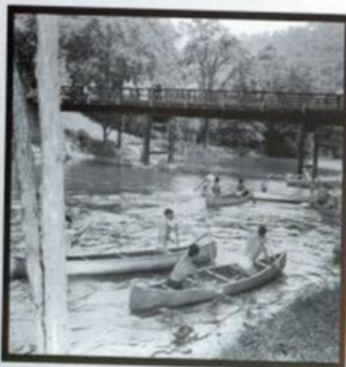
▲ One more shot of Sherman's Creek and the wooden decked bridge that was erected in 1949, to provide year-round access to the Loyville Scout Camp through the East Gate. The steel support was designed and furnished to the Council by Bethlehem Steel Company. The wood deck and railing was replaced in 2001.
