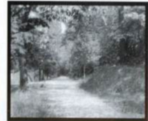
Above - This photo was marked "The Company Street." The road may have served as a camp entrance. The camp was connected to Harrisburg by the Pine Grove Furnace branch of the P&R (Reading) Railroad.
