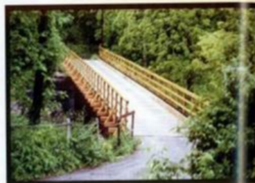
▲ As part of the renovations of the Hidden Valley Scout Reservation, the original wood/steel bridge over Sherman's Creek is having a new deck installed in this scene. The old wooden deck has already been removed and the crew is now installing new oak timbers beginning at the east end. Vehicles can be seen parked on the Rotary parking lot at the far left in back of the trees. The steel work was designed and supplied by Bethlehem Steel Company many years ago. This photo was taken in March, 2000. Photo courtesy of Sharon Lance
