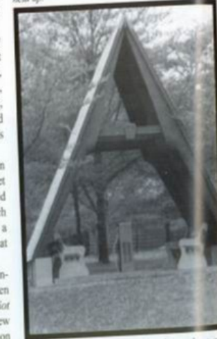
The Memorial A-Frame building, shown above, was built as a common meeting place and dedicated to the memory of William "Bill" Dowling. Construction was under the direction of Charlie Steele, and in typical Steele style, the rafters were made from government surplus whale boat keels, donated by the Mechanicsburg Naval Supply Depot. While under construction, the workers affectionately called the building "Charlie's Car Wash."
