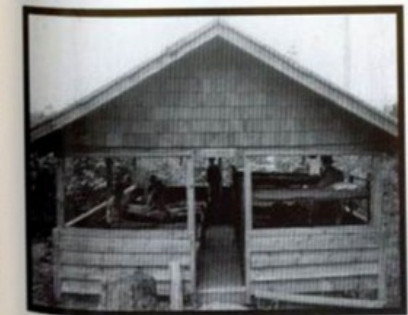
Below - This is one of the permanent camping structures constructed in Hidden Valley. Each building could house eight single cots, many used double bunks, as shown here. The sign above the door reads, "Materials for this shack furnished by R. H. Appleby. Construction by Scouts and Leaders."
