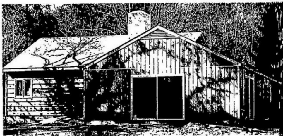
LEADERSHIP DEVELOPMENT BUILDING Opened in 1979 at Ockanickon.
