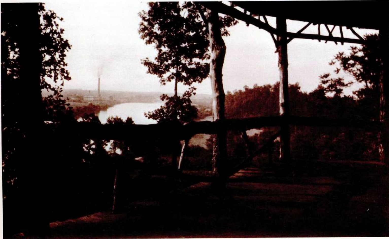
Camp McDonald from the cabin veranda, looking north at the Southern Power Utilities steam plant on the Catawba River, left.
