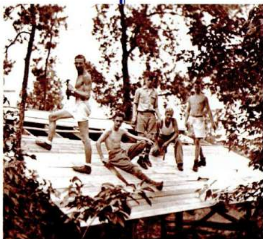
Troop 11 Scouts building a roof on a shelter.
