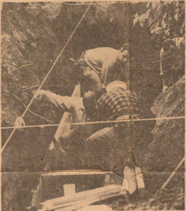
DEEP DIGGERS . . . Utica area Seabees went deep yesterday as they laid the foundation for a new lodge room at Camp Russell.
