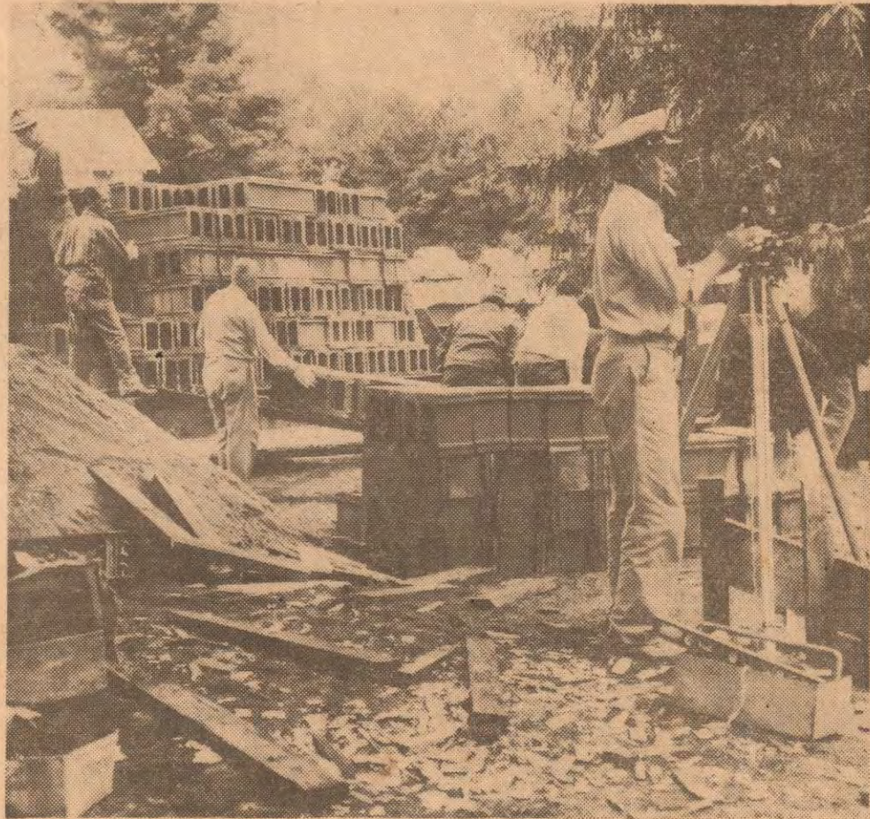
VOLUNTEERS AT WORK . . . Camp Russell, White Lake, took on the appearance of a battlefront construction scene of World War II yesterday as the local Seabees moved in to work for a weekend on new buildings at the scout camp. (Photos by Dante Tranquille.)
