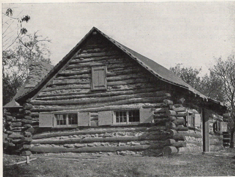
LOG CABIN BUILT BY BOY SCOUTS OF WAYNE
