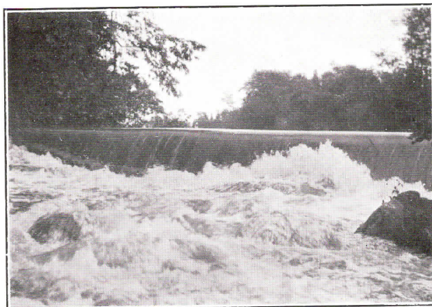
DAM AT CAMP DELMONT
