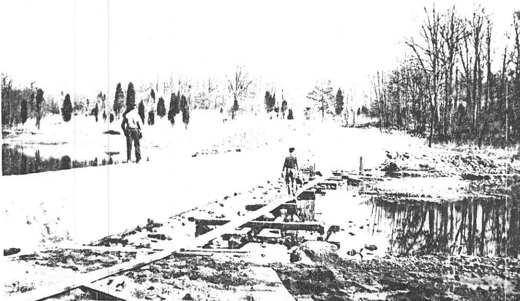
Dam under Construction Unami Creek 1934 - cost of $20,000
